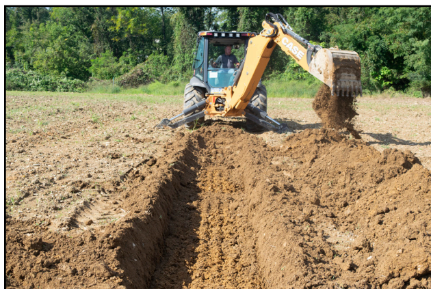
Figure 9: Backhoe stripping in the Wiest lower field (Photo number 2021_D_056)
