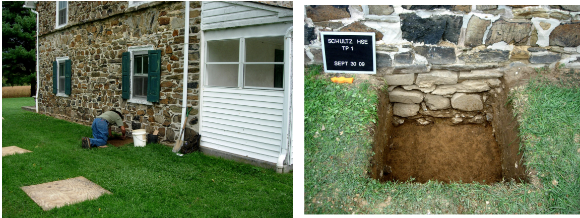
Figures 24a-b. TP1 excavation in progress, facing northeast (left); TP1 excavation completed, facing east (right).
